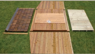
2. LAY OUT PRE-MADE PANELS
