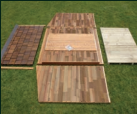
LAY OUT PRE-MADE PANELS
